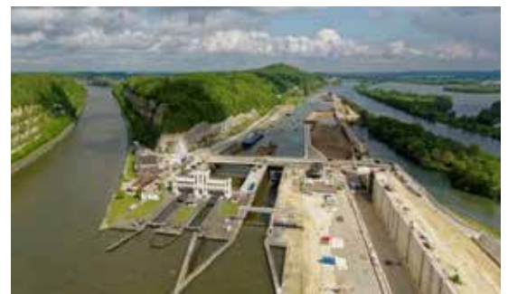
Lanaye Lock #4 being constructed
